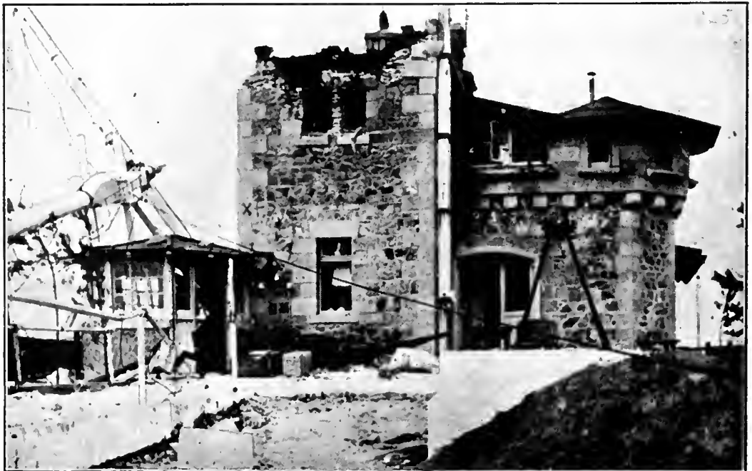
TSING-TAU WIRELESS STATION DESTROYED.
